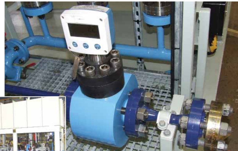
Left: Litre Meter has supplied VFF meters to Geveke Pompen used to monitor MEG which helps prevent hydrate formation in lines on the new Wingate natural gas well in the North Sea
