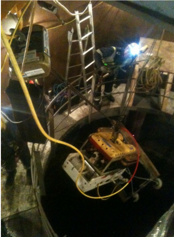
Launching ROV Integrated Scanner within the Monopile.
