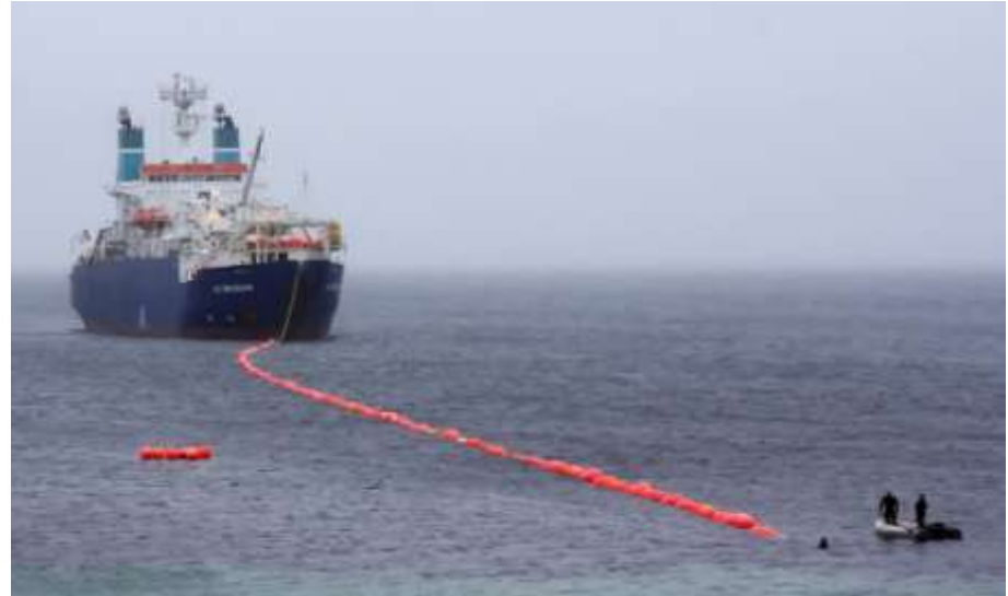
Cable installation at EMEC – Falls of Warness. Image Courtesy of EMEC
